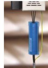
CoolTUBE® installed on VFD leads to servo
