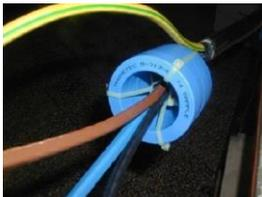
CoolBLUE® installed on leads between VFD and servo
